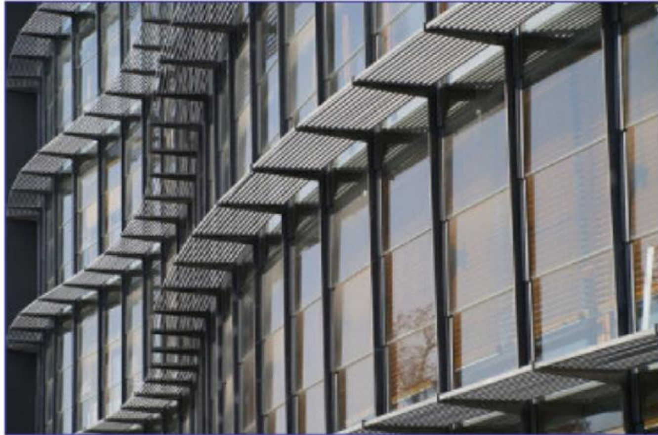
Example of passive façade: The Moravian Library in Brno (Czech Republic) [77].
