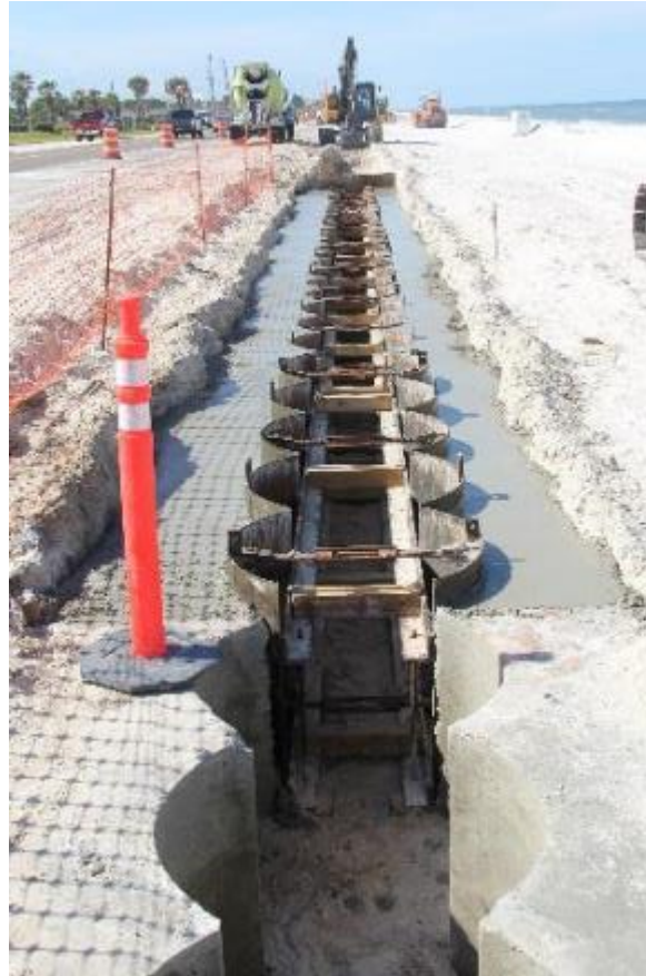
Secant-piles installed via guide wall form
